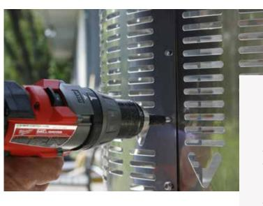
Start screws in three of the holes in the top half of the incinerator. The 10-32x1/2" self-threading S.S. screws must be inserted from the outside but should not be completely tightened at this time. Do not place screws in the 1st and 2nd holes from the top or the last hold from the bottom as these will be used later for the Base Ring and Cover Clips. Follow the above procedure to assemble the third and fourth panel, forming a cylinder.
